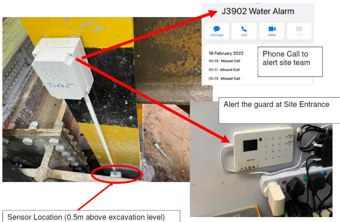
Figure 21 Water Detection Sensors
