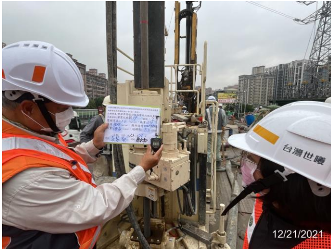
Figure 5. The Inspection of rod lift (Jet grouting method)
