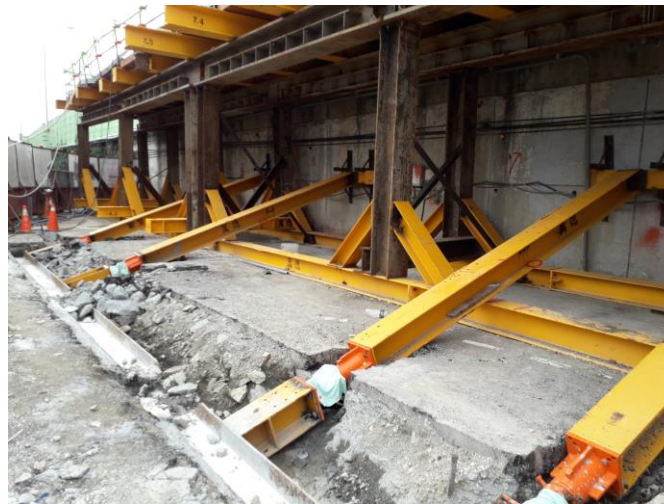
Figure 10. Retaining wall with added lateral support to control displacement
