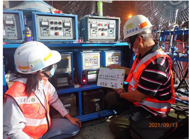
Figure 6. The Inspection of grout flow rate and pressure (Double packer method)
