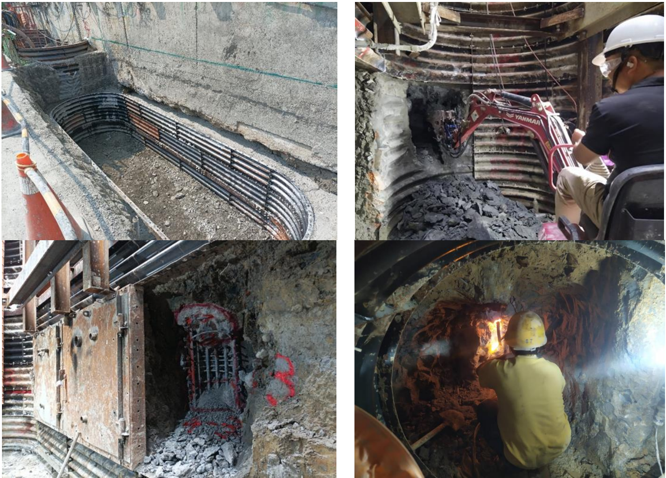
Figure 13. The photo of the foundation pile removed
