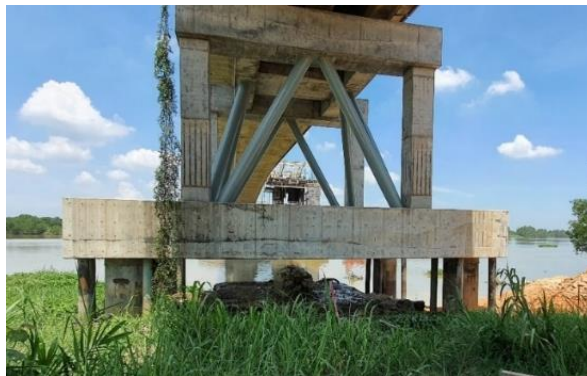
Figure 21. Completed Restoration of Pier 11
